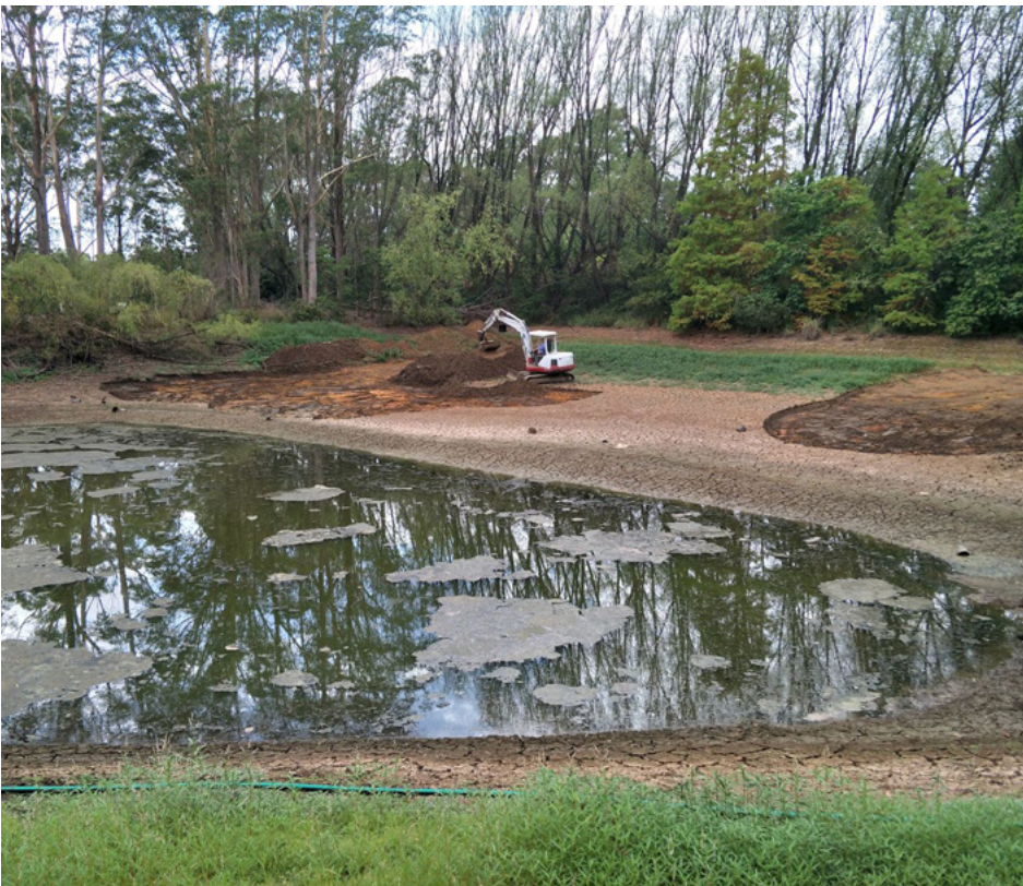
Building a new dam, Engall's Nursery, NSW.
