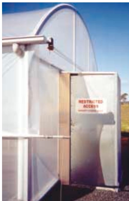
Restricting access of staff and visitors is required to maintain hygiene. Advantage Plant Production Nursery, NSW.
