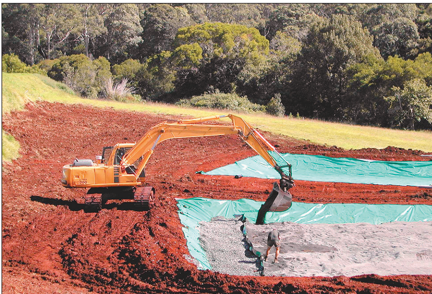
Bau Farm Wholesale Nursery on the New South Wales north coast has a production area of five hectares. To clean its runoff water two reed beds were constructed, each 150 cubic metres, sealed with heavy-duty plastic and filled with five millimetres of blue gravel.
