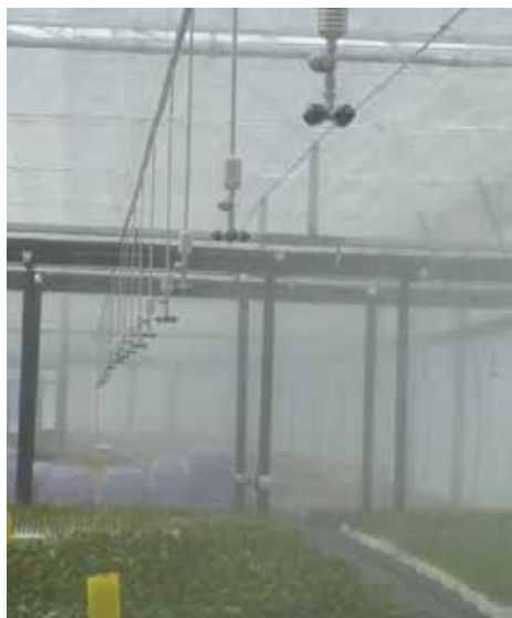
An effective inline fogging system to control humidity in a propagation area with misters (hanging) at Native Plant Wholesale Nsry (BioSecure HACCP)
