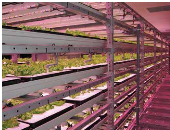
Fig 4. LEDs maximising space with multilayering Source: Phillips Australia
