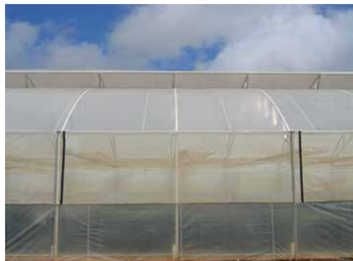
A modern greenhouse with high side walls, roof ventilation, internal screens and the ability to deliver good light levels for plant growth - NIASA accredited Alstonville Palms, NSW
