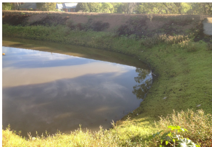
Management of the recirculated water storage to restrict potential for weed growth is paramount to reducing organic matter and weed seeds which can deprive oxygen levels and facilitate production of hydrogen sulphide.
