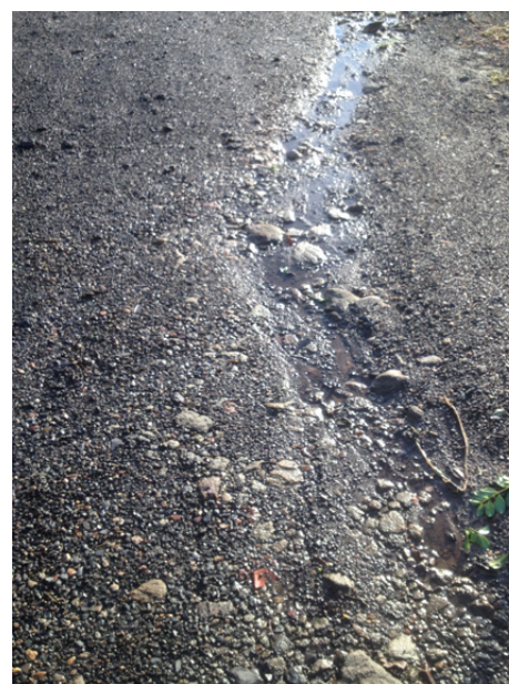
Consider how runoff generated within a nursery is dealt with. In this instance no clear drainage plan allows runoff to flow over roads and paths which is either lost due to evaporation and seepage or to collect sediment.
