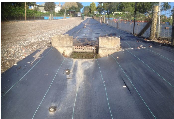
Drainage works do not need to elaborate, just effective in collecting runoff, retarding speed and removing sediments before directing to a water storage (courteous Engalls Nursery)
