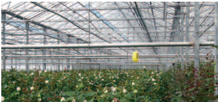
While glass provides better light transmission than most plastic options, its heavier weight requires more substantial structures resulting in shadows that may affect the crop.
