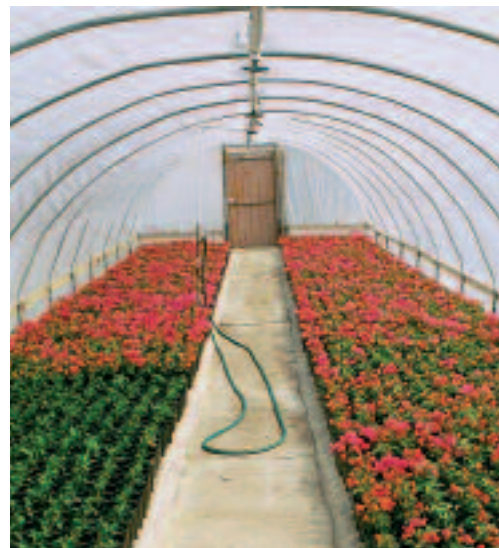
Low technology greenhouses are relatively cheap and easy to build. However, they offer minimal control over the growing environment.
