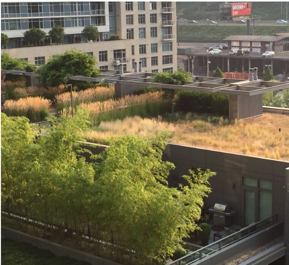
The number and area of green roofs in Australia is low compared to other countries, for example some states in the USA, where green roofs are encouraged, and sometimes mandated, through a range of policies. Image: N Williams.
